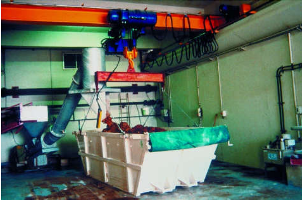
Figure 292. Screenings press.
