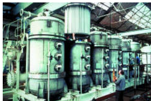
Figure 63. A Shell facility in Brent (North Sea). Flow: 2100 m 3 .h -1 . Precoat filters.
