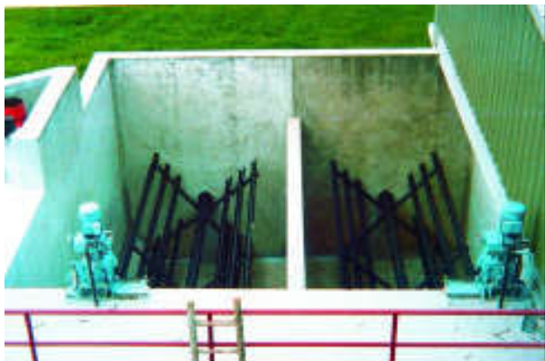
Figure 300. Paddle type flocculator.
