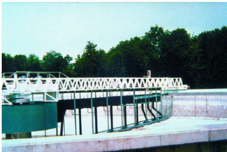
Figure 324. Mulhouse (Eastern France) facility. Flow: 98,135 \text{ m}^3 \cdot \text{d}^{-1} . SRP-type settling tank.
