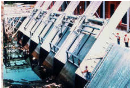
Figure 269. Rack and pinion bar screens.
