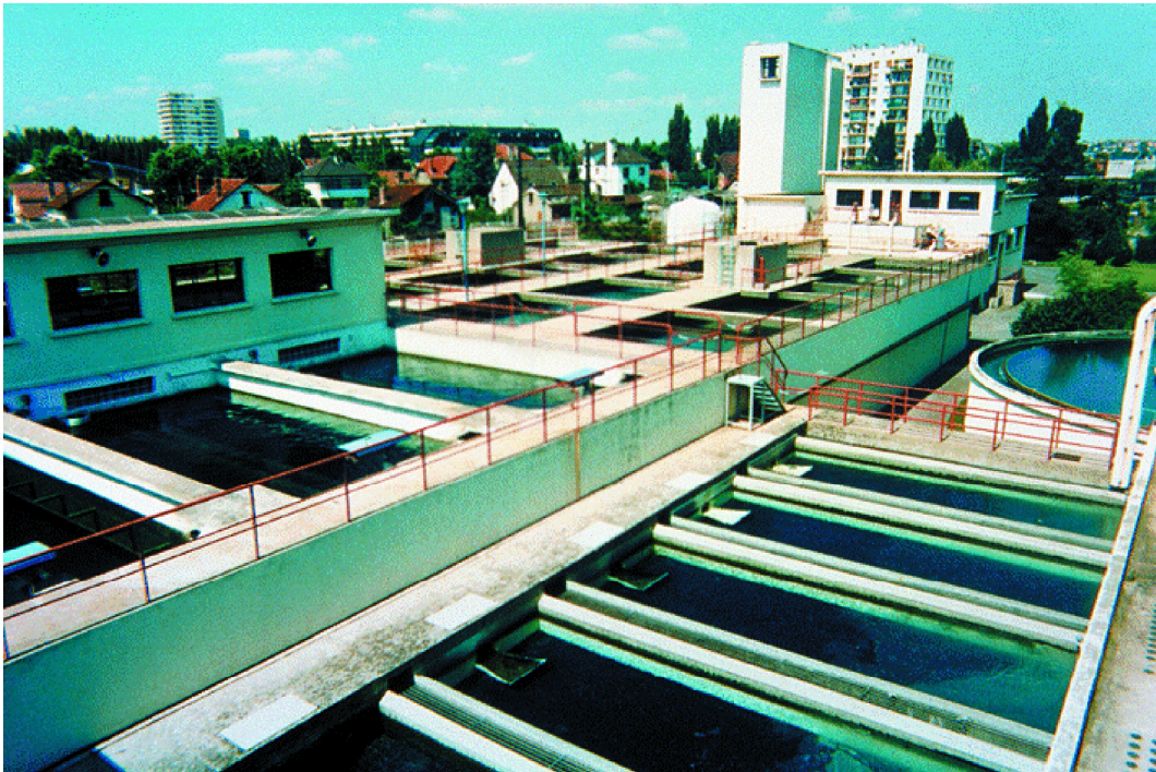
Figure 98. Vity-Chdtillon facility, Paris area (France) - LE-Dumez. Flow: 4,000 \text{ m}^3 \cdot \text{h}^{-1} . 6 Mediazur T filters and 9 Mediazur V filters.
