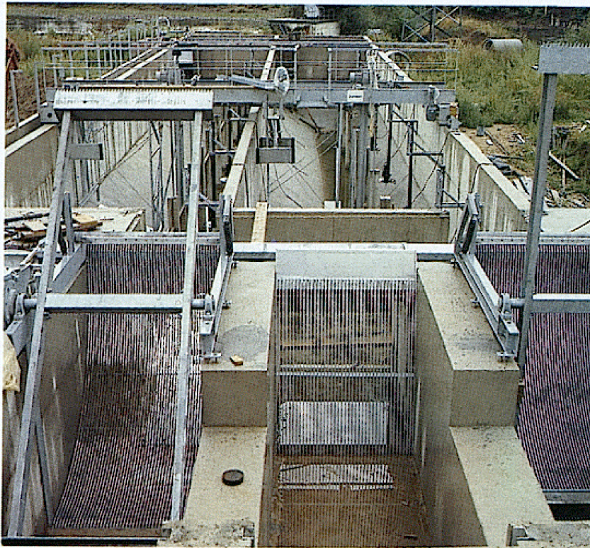
Figure 264. Curved bar screen (DC type).
