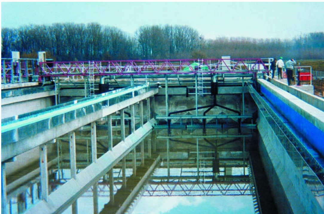
Figure 329. Strasbourg (Eastern France) facility. Flow: 242,000\text{ m}^3 \cdot \text{d}^{-1} . SLG-type settling tank. 18 units, 20\text{ m} \times 66\text{ m} each.
