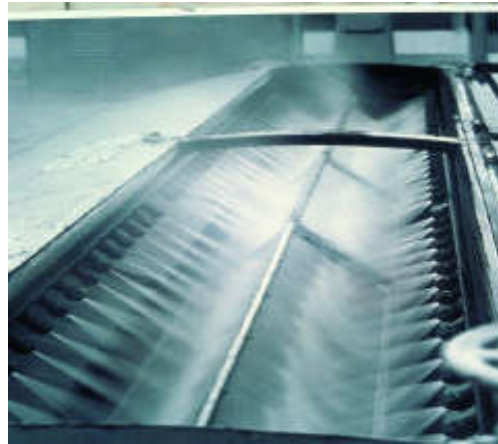
Figure 60. Microstrainer with dihedral filtering elements. Washing the filter cloths.
