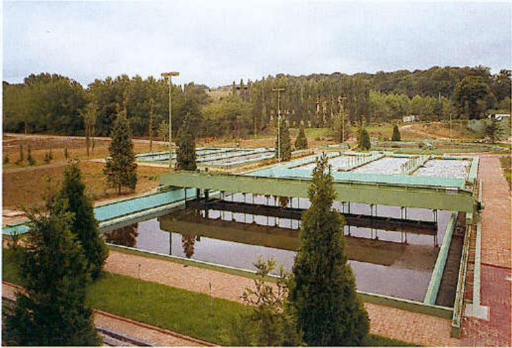
Figure 330. La Minière (Paris area, France) facility. Flow: 12,000 \text{ m}^3 \cdot \text{d}^{-1} . Cross-flow settling tank, 21 m x 29.5 m.
