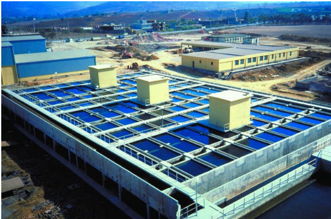
Figure 335. Boudouaou facility for drinking water supply for Greater Algiers (Algeria). Flow: 540,000 \text{ m}^3 \cdot \text{d}^{-1} . Surface water clarification. Six Pulsatube clarifiers. Unit area: 551 \text{ m}^2 .
