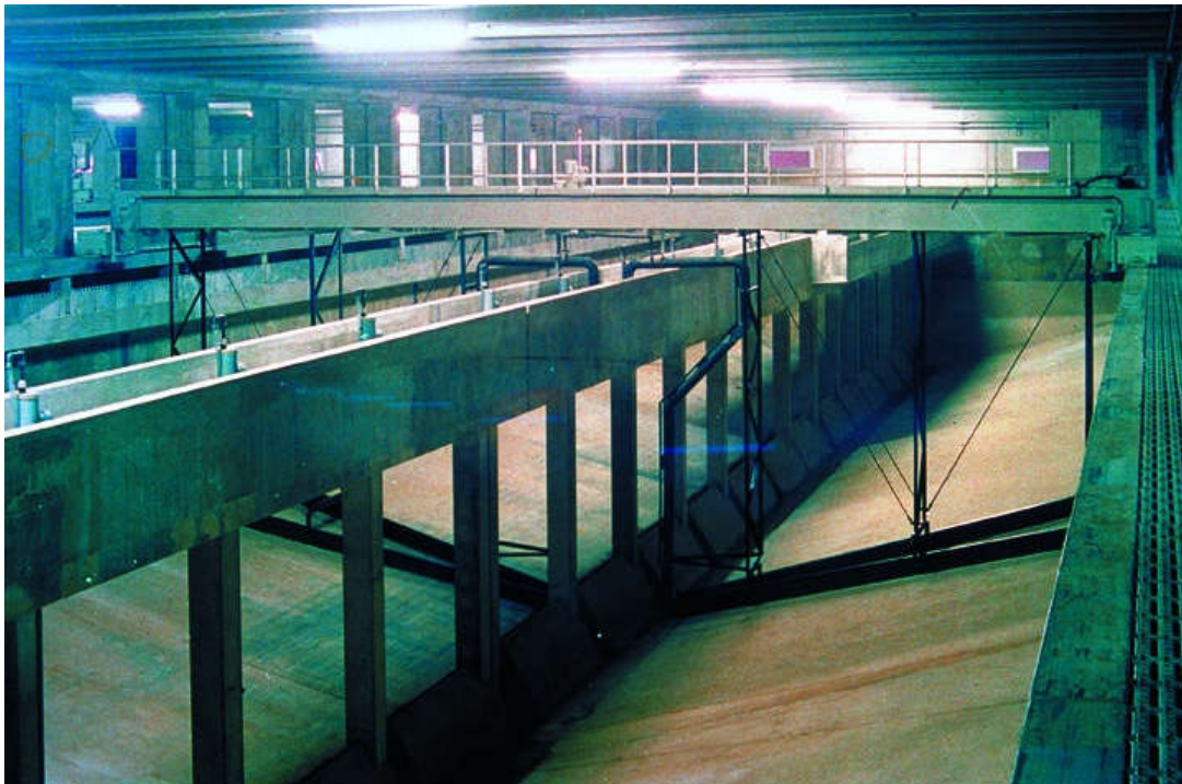
Figure 331. Nice (Southern France) facility. Flow: 220,000 \text{ m}^3 \cdot \text{d}^{-1} . One of 12 secondary clarifiers, 15 m x 60 m.
