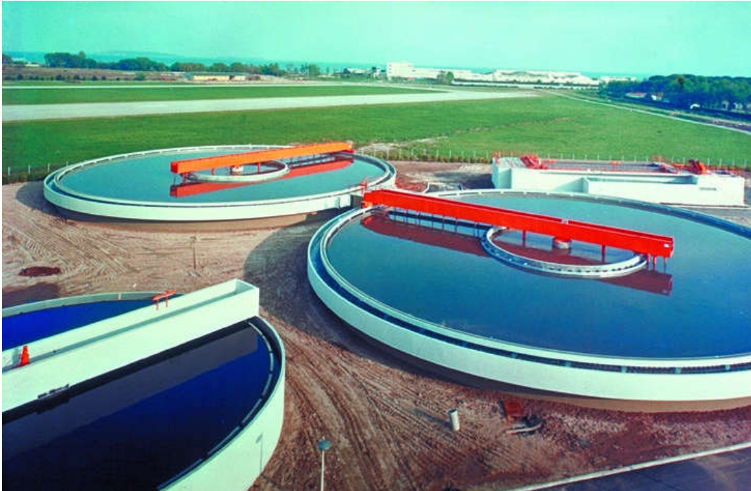
Figure 310. Cannes (Southern France) facility. Maximum flow: 5,500 \text{ m}^3 \text{ h}^{-1} . Flocculator/settling tanks.
