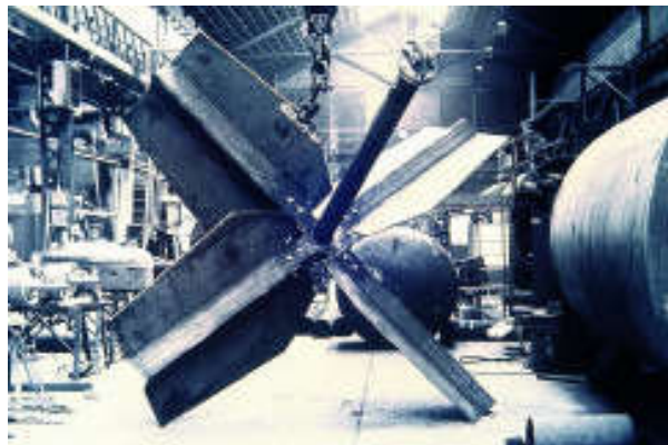
Figure 301. Propeller type flocculator.
