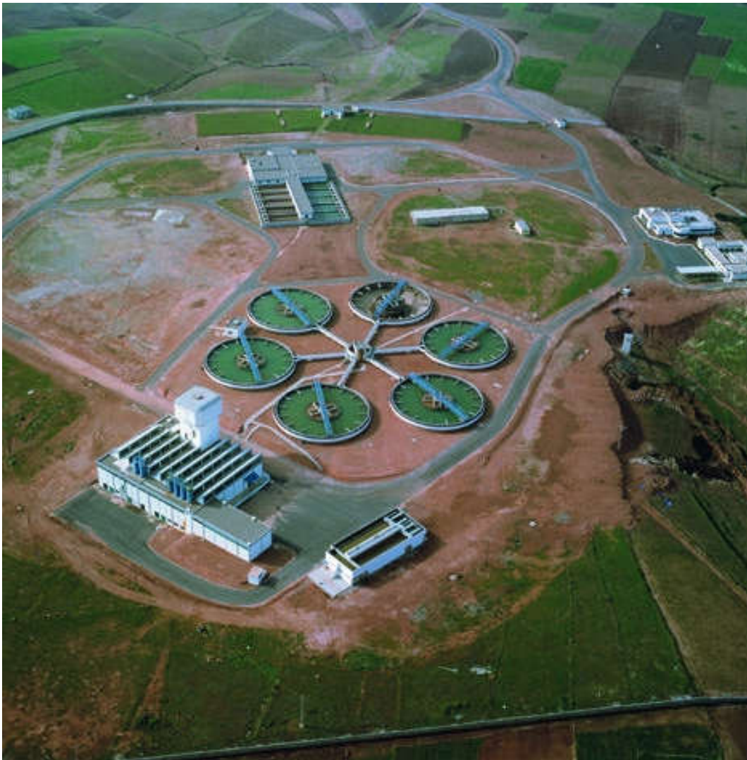
Fig. 275. Circular scraper settling tanks for presedimentation.
