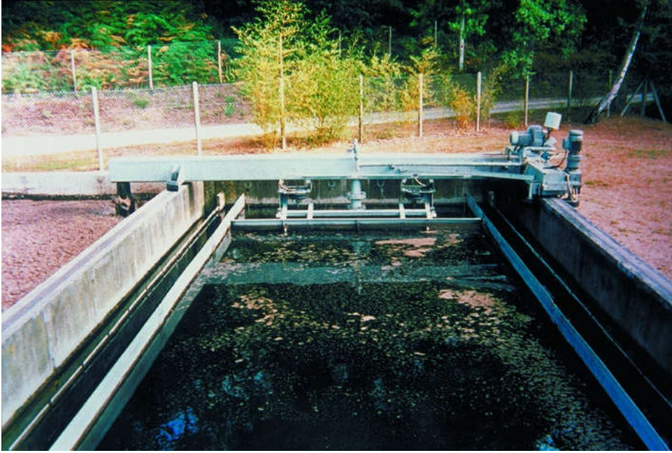
Figure 395. Compact MA with a rectangular settling tank.
