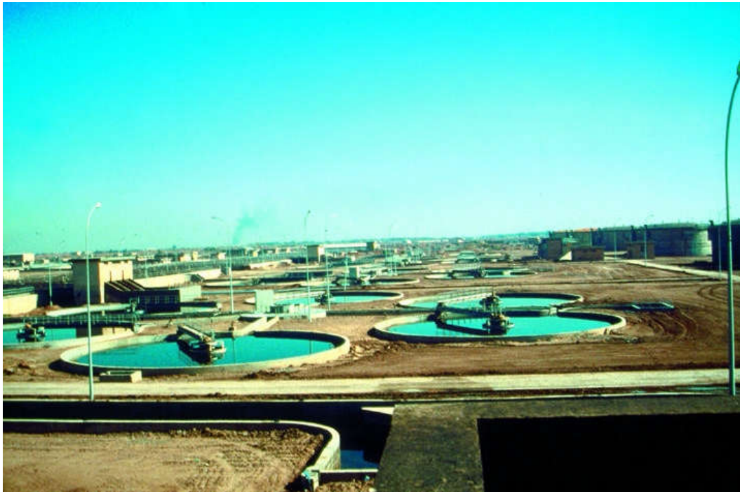
Figure 304. Facility in Kerkh (Iraq). Capacity: 1,200,000 PE Primary settling tanks.
