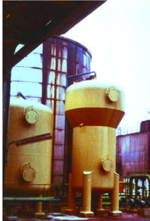
Figure 464. Treating oily condensates. Capacity: 90 \text{ m}^3 \cdot \text{h}^{-1} .
