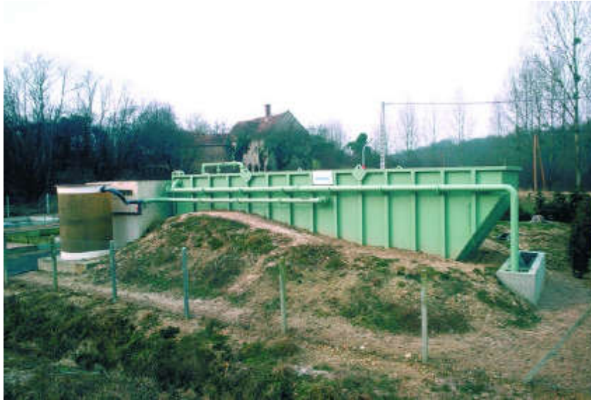
Figure 393. Dampierre-en-Burly facility, France. Capacity: 400 population equivalents. Minibloc AP.
