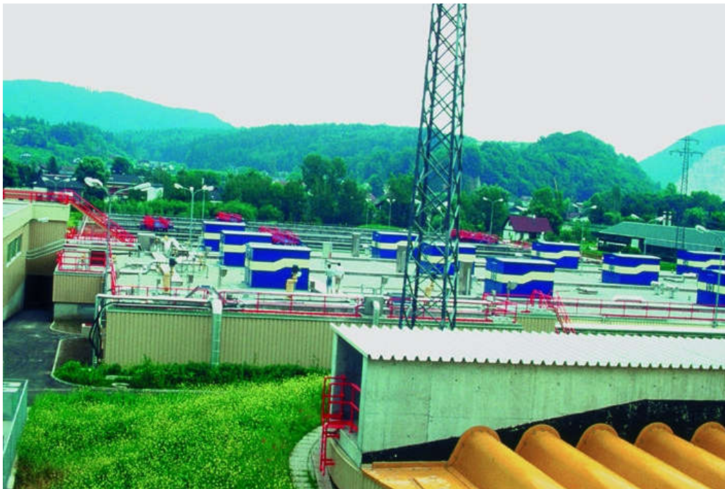
Figure 391. Leykam plant Austria. Treatment of paper mill effluents. Flow: 856M 3 h -1 . Pure oxygen activated sludge reactor.
