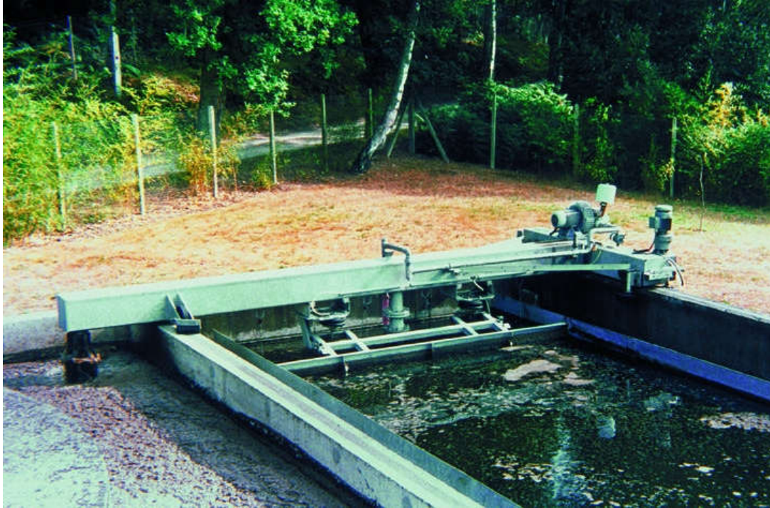
Figure 328. SLP-type settling tank,
