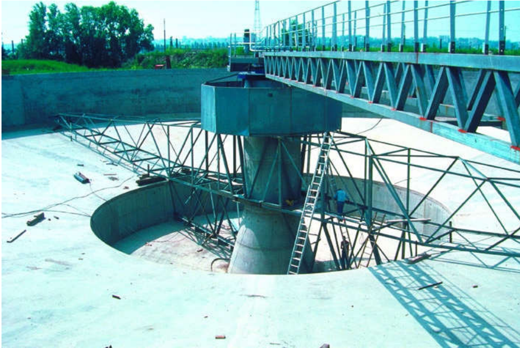
Figure 308. Valenton (Paris area, France) facility for SLUR Flow: 300,000\text{M}^3 \cdot \text{d}^{-1} , Central drive unit on the concrete centre column of a primary settling tank, 52 m dia.
