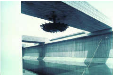
Figure 375. 75 kW R 8020 Actirotor installed on a reinforced concrete walkway.
