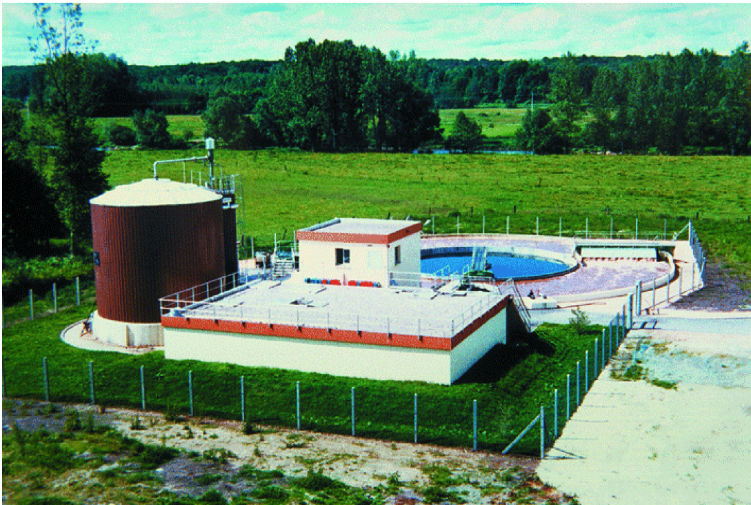
Figure 153. The Anafix fixed bed reactor. The Saint-Hubert dairy. Magnieres factory in eastern France.
