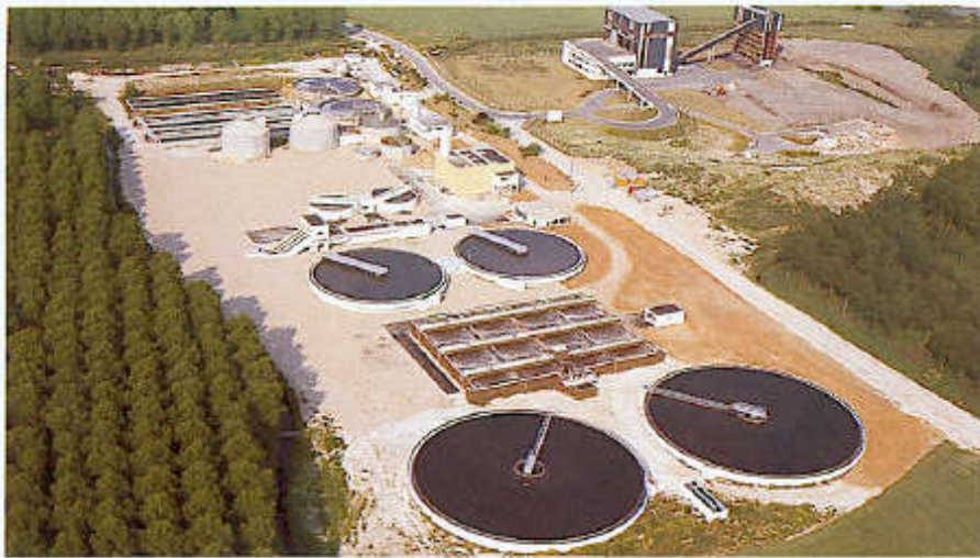
Figure 377. Reims plant, France. 5,250 \text{ m}^3 \cdot \text{h}^{-1} . Biological purification of MWW by activated sludge. 2 tanks each 3,750 \text{ m}^3 and equipped with six 37 kW R 6016 Actirotors.
