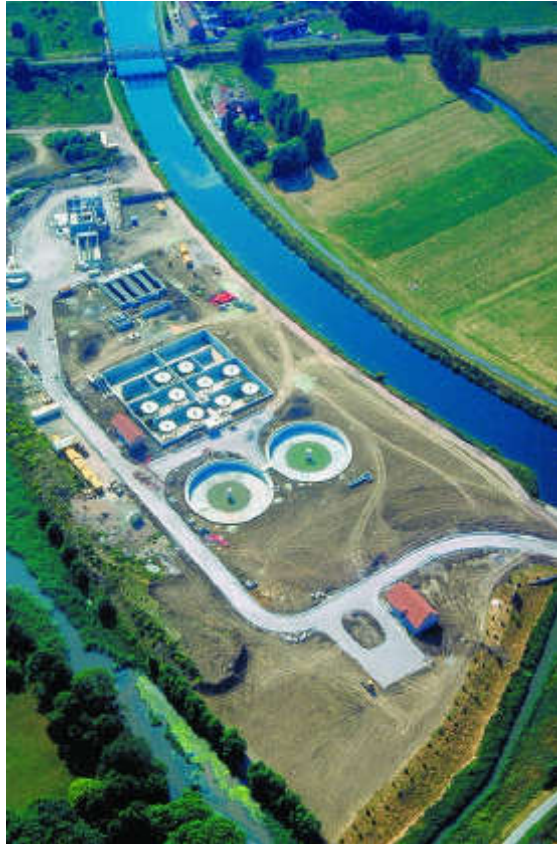
Figure 323. Ploegsteert-Comines (Belgium) facility. Flow: 22,650 \text{ m}^3 \cdot \text{d}^{-1} . Aerial view of SR-type settling tanks.
