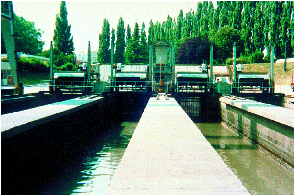
Figure 263. Back-cleaned screen installation.
