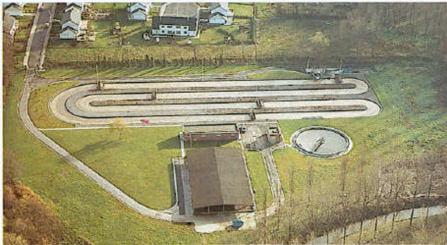
Figure 397. Waremme plant, Belgium. Oxidation ditch with Rollox for MWW treatment.
