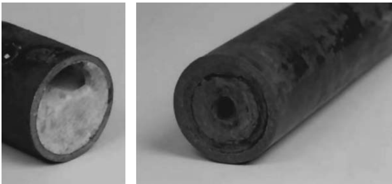
FIGURE 1.2 Boiler scale deposits formed on the water side.
