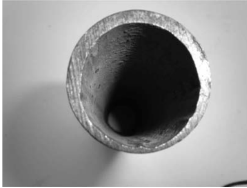
FIGURE 15.6 Carbonic acid corrosion. (Courtesy of Guardian CSC, York, Pennsylvania.)
