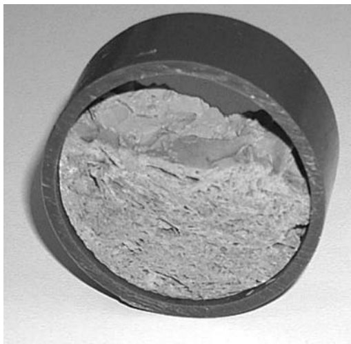
FIGURE 1.7 Cemented calcium carbonate deposits formed in a PVC drinking water transport pipe.
