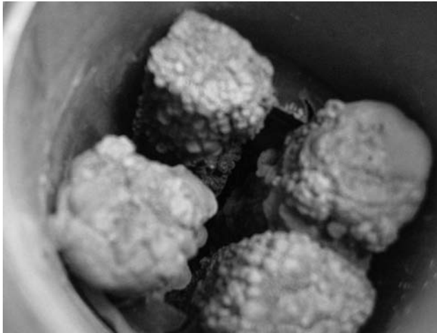
FIGURE 20.3 Pipe corrosion due to hyperchlorination.
