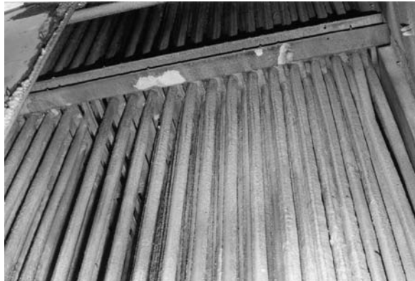
FIGURE 1.6 Calcium carbonate deposits in an ammonia cooling tower.
